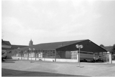
Remise (ancienne usine U.M.D.). Phot. Laurent Poupard IVR43_19893900208Z
