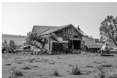
Façade postérieure. Phot. Gilbert Poinot IVR43_19752500784Z
