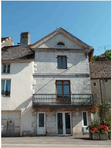
Vue nord Phot. Sabrina Dalibard IVR43_20137000798NUC2A
