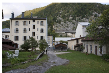
Elévation postérieure. Phot. Yves Sancey IVR43_20093900128NUC2A
