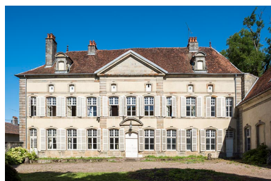
Façade principale. Phot. Sonia Dourlot IVR43_20167001147NUC4A
