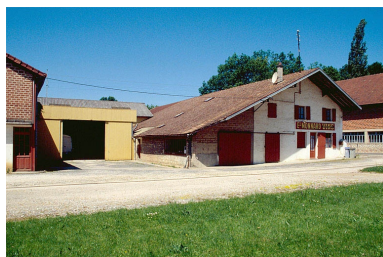
Magasin industriel. Phot. Jérôme Mongreville IVR43_19963900445ZA
