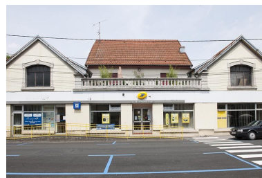
Vue de face. Phot. Jérôme Mongreville IVR43_20112501607NUC4A
