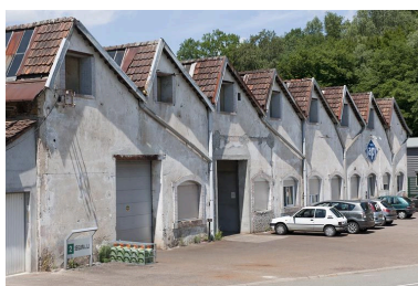
Atelier de fabrication des pompes. Sheds est. Phot. Jérôme Mongreville IVR43_20112501182NUC4A
