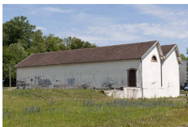
Magasin industriel est. Phot. Jérôme Mongreville IVR43_20112501186NUC4A
