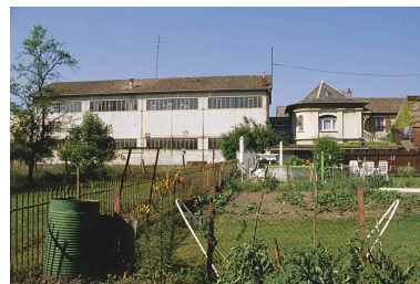
Façades nord. Phot. Yves Sancey IVR43_20009000538ZA
