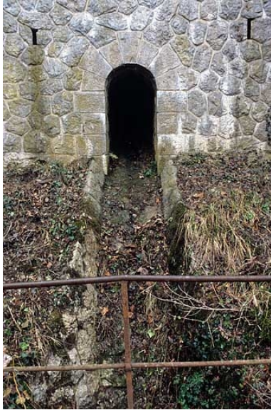
Aqueduc de 70 cm. Phot. Yves Sancey IVR43_20053900666ZA
