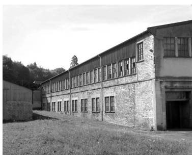
Atelier de fabrication est. Phot. Jérôme Mongreville IVR43_19973901074X
