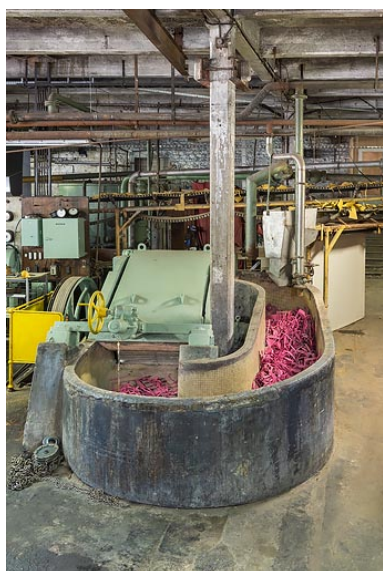
Pile raffineuse. Phot. Pierre-Marie Barbe-Richaud IVR43_20203900103NUC4A
