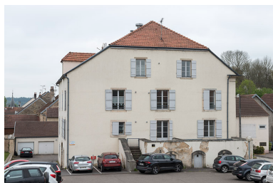
Façade est. Phot. Jérôme Mongreville IVR43_20177000721NUC4A
