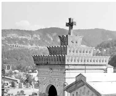
Toiture. Phot. Yves Sancey IVR43_20033901084X
