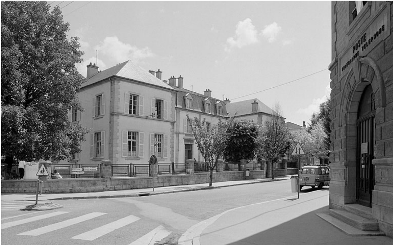
Ecole, 1 avenue Aristide Briand, façade antérieure.
