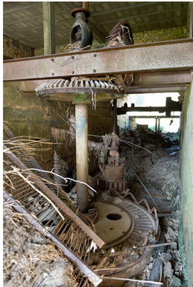
Moulin : turbine Pougnet. Phot. Sonia Dourlot IVR43_20182501765NUC4A
