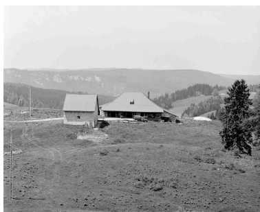
Vue de situation. Phot. Yves Sancey IVR43_19993900107X
