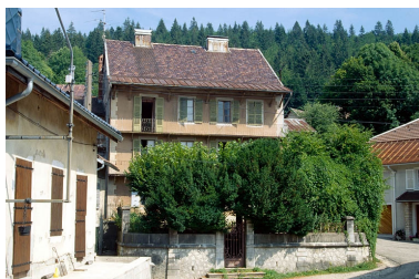
Logement patronal. Phot. Laurent Poupard IVR43_19913901605ZA
