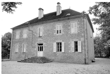
Logement patronal. Phot. Jack Dumont IVR43_19803900341Z
