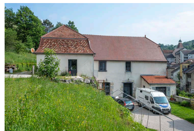
Façades sud. Phot. Jérôme Mongreville IVR43_20233900396NUC4A
