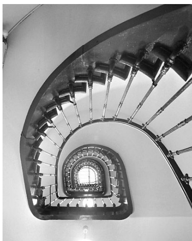
Escalier. Phot. Yves Sancey IVR43_20033900726X
