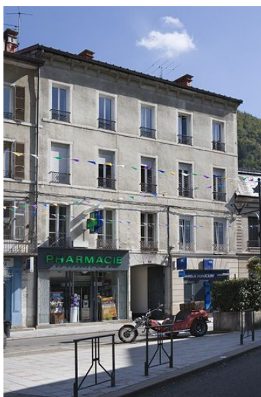
Façade antérieure. Phot. Yves Sancey IVR43_20093900149NUC2A
