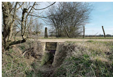
Aqueduc. Phot. Jean-Luc Duthu
