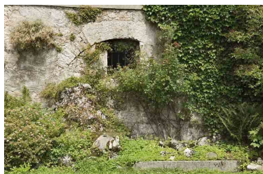
Citerne. Phot. Jérôme Mongreville IVR43_20092501140NUC2A
