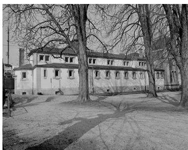
Aile orientale (1983). Phot. Yves Sancey IVR43_19833900097X
