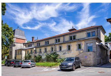
Aile occidentale. Phot. Jérôme Mongreville IVR43_20223900771NUC4A
