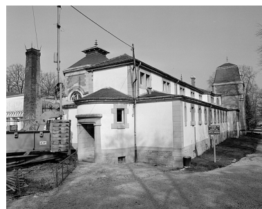
Aile orientale (1983). Phot. Yves Sancey IVR43_19833900096X
