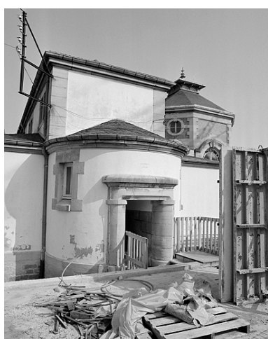
Aile orientale (1983). Phot. Yves Sancey IVR43_19833900095X
