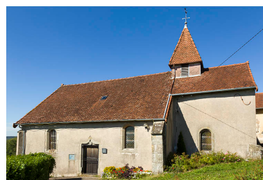
Façade sud. Phot. Sonia Dourlot IVR43_20157000534NUC2A
