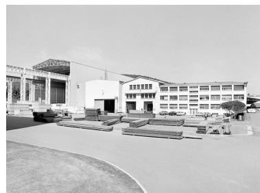
Atelier de fabrication (emballage). Phot. Jérôme Mongreville IVR43_20029000131X
