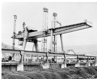
Pont roulant. Phot. IVR43_20029000220X
