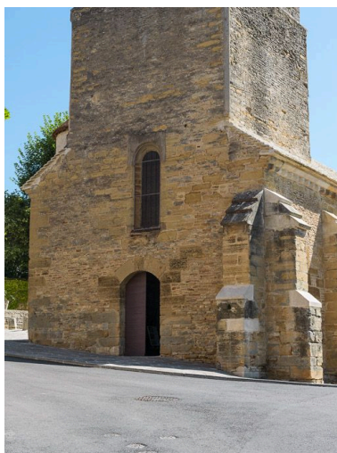
Façade. Phot. Pierre-Marie Barbe-Richaud IVR26_20162100430NUC2A
