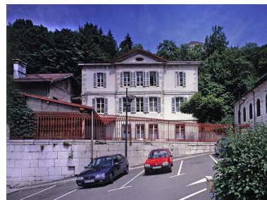
Façade antérieure. Phot. Yves Sancey IVR43_20033900824VA
