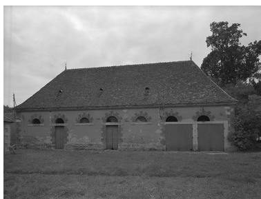
Ecuries. Phot. non renseigné IVR26_19755800536V
