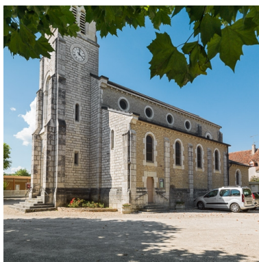
Elévation est. Phot. Pierre-Marie Barbe-Richaud IVR26_20162100277NUC2A
