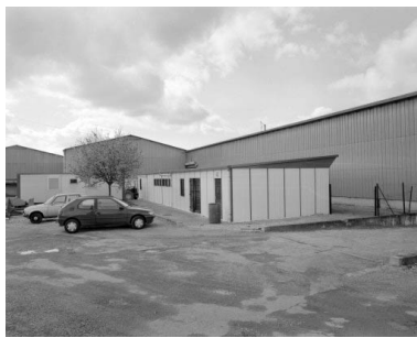
Bungalow (A). Phot. Yves Sancey IVR43_19943901651X
