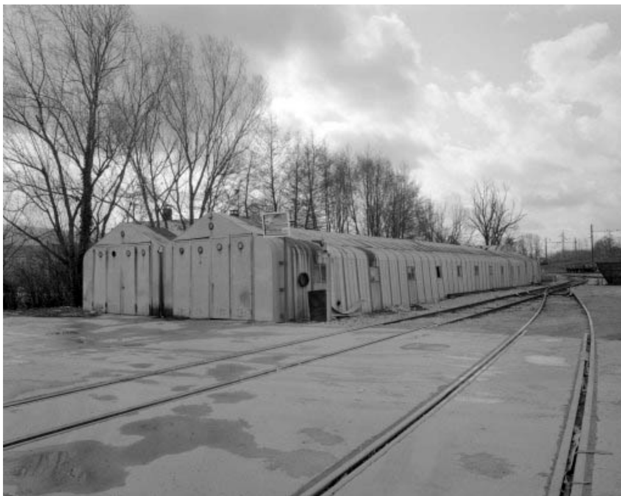
Baraques de chantier (F).
