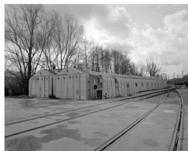
Baraques de chantier (F). Phot. Yves Sancey IVR43_19943901660X
