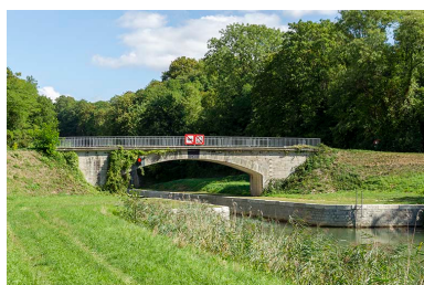
Pont routier en aval du tunnel. Phot. Sonia Dourlot IVR43_20167001843NUC2A
