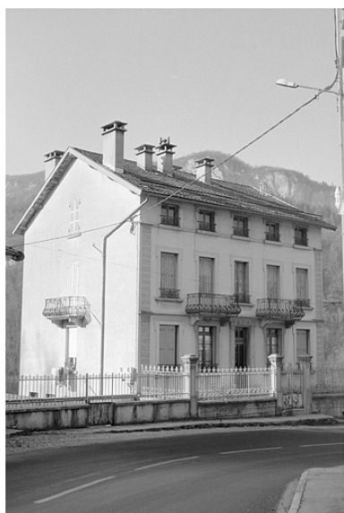
Logement patronal. Phot. Laurent Poupard IVR43_19913901131Z
