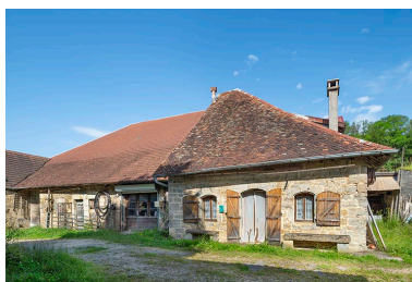
Façade est. Phot. Jérôme Mongreville IVR43_20243900735NUC4A
