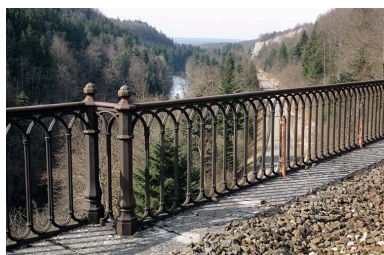
Garde-corps. Phot. Yves Sancey IVR43_20053900101ZA
