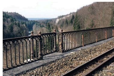
Refuge et garde-corps. Phot. Yves Sancey IVR43_20053900103ZA
