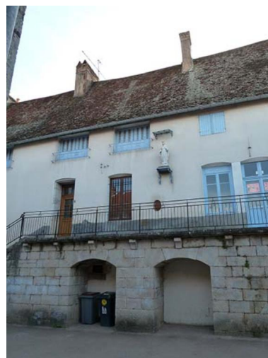
Façade nord Phot. Sabrina Dalibard IVR43_20137000822NUC2A
