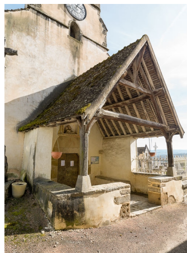
Porche. Phot. Pierre-Marie Barbe-Richaud IVR26_20177100106NUC2A
