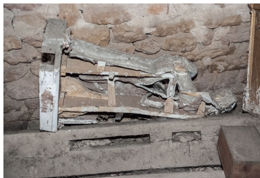
Combles. Phot. Pierre-Marie Barbe-Richaud IVR26_20177100120NUC2A
