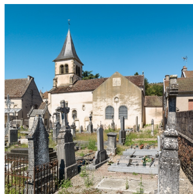
Elévation sud. Phot. Pierre-Marie Barbe-Richaud IVR26_20167100062NUC2A
