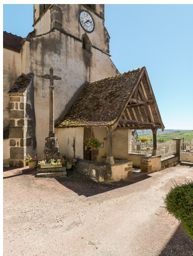
Porche. Phot. Pierre-Marie Barbe-Richaud IVR26_20167100060NUC2A
