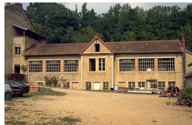
Atelier de fabrication. Phot. Laurent Poupard IVR43_19913901103ZA
