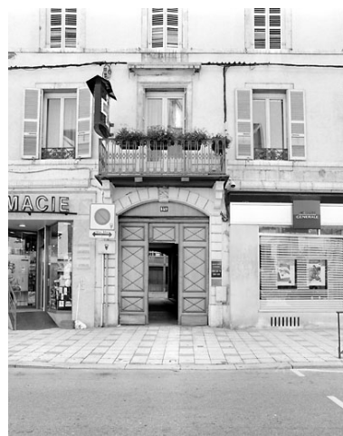
Entrée principale. Phot. Yves Sancey IVR43_20033900734X
