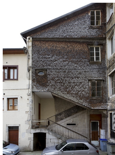
Escalier sud. Phot. Yves Sancey IVR43_20103900445NUC2A
