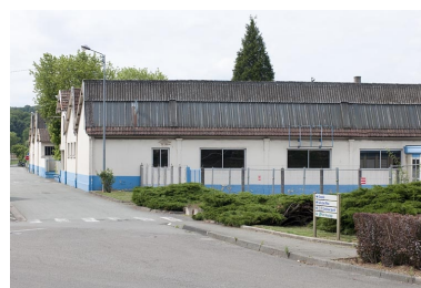
Ateliers de fabrication originels.
