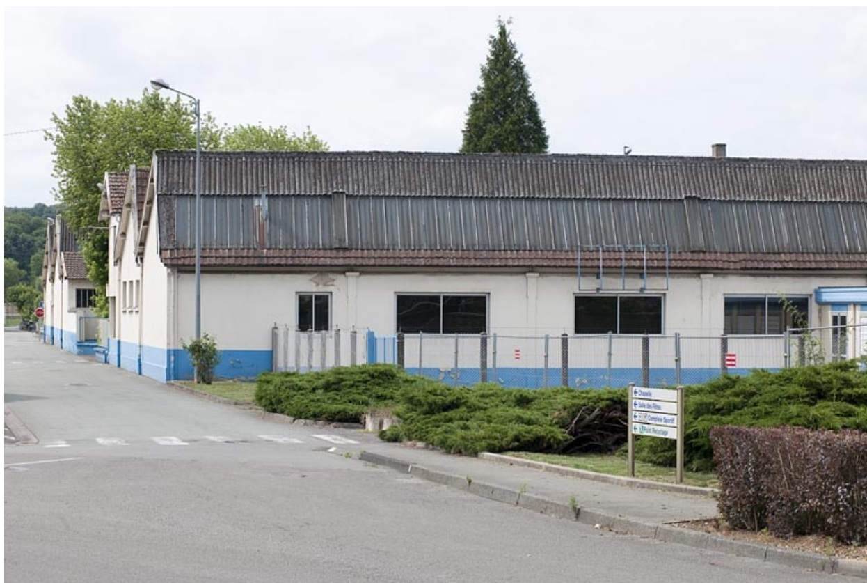
Ateliers de fabrication originels.
