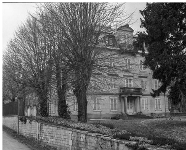
Façade principale. Phot. Jérôme Mongreville IVR43_19853900140X
