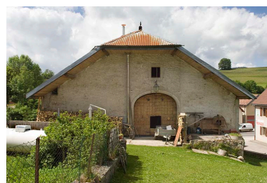
Façade postérieure. Phot. Jérôme Mongreville IVR43_20092500787NUC2A
