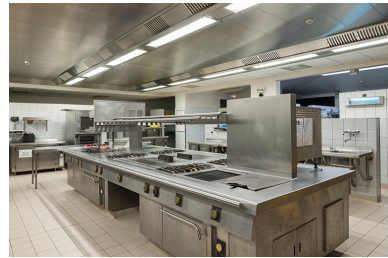
Cuisine du restaurant d'application. Phot. Jérôme Mongreville IVR43_20142500467NUC4A
