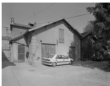
Remises. Phot. Jérôme Mongreville IVR43_19973900275V
