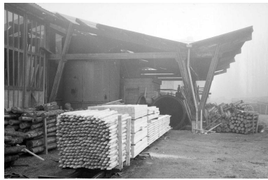
Autoclave. Phot. Laurent Poupard IVR43_19893900277Z
