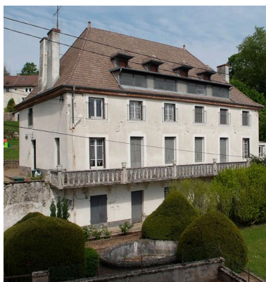
Moulin : habitation. Phot. Jean-Luc Duthu IVR26_20107100403NUC2A
