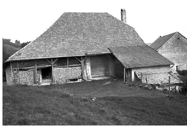
Façade postérieure. Phot. Gilbert Poinot IVR43_19762500946Z
