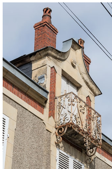
Lucarne portant la date ("1883"). Phot. Pierre-Marie Barbe-Richaud IVR26_20205800462NUC4A
