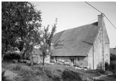
Façade postérieure. Phot. Michel Rosso IVR26_19852101090V
