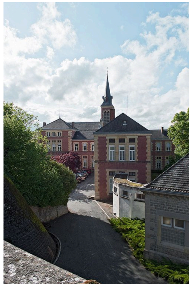
Elévations sud-est. Phot. Pierre-Marie Barbe-Richaud IVR26_20107100779NUC2A
