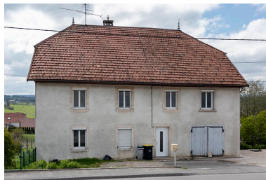
Façade antérieure. Phot. Sonia Dourlot IVR43_20192500382NUC4A
